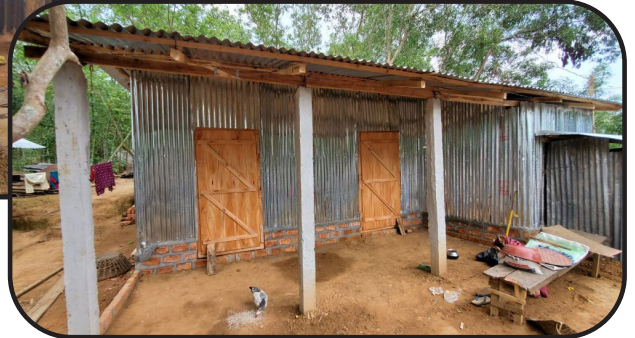
After: A secure residence in progress!
